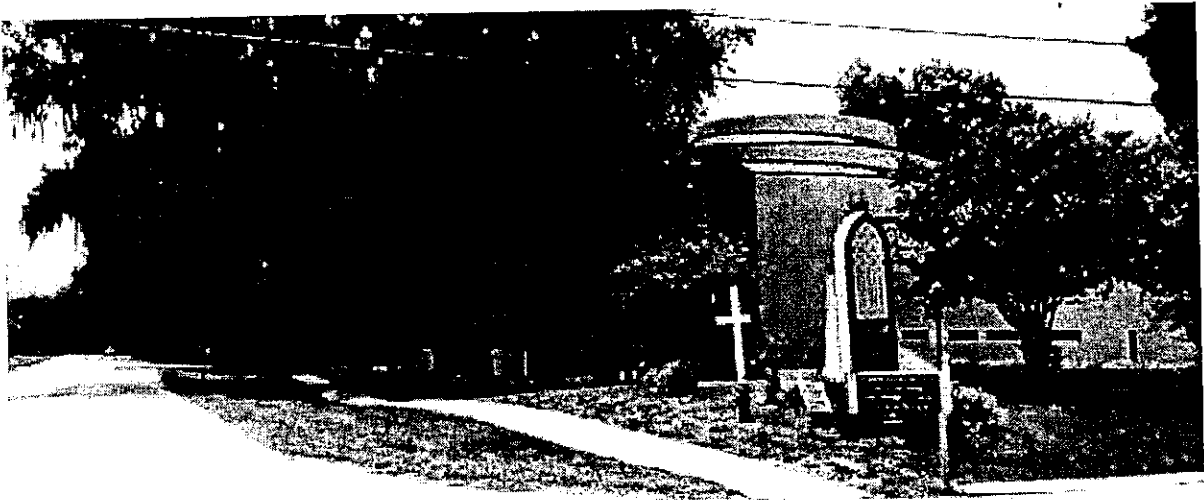
Facing south along Ft Caroline Rd with the subject site/sign on the right
